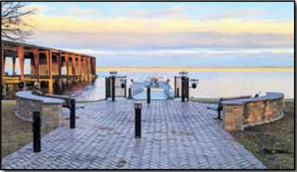
New: Village dock with 200' water and electric hook-ups, up to a 72-hour stay!
